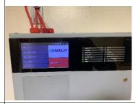
The previous fire risk assessment raised an action that the EACIE alert system was sounding with a fault at the time of the FRA. At the time of the fire risk assessment the panel was free from faults, this action has been completed.
