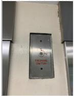
A new Evacuation Alert System (EACIE) has been installed within the building. The EACIE is equipped with facilities for use by the Fire and Rescue Services (FRS), enabling them to send an evacuation signal to the whole or a selected part of the building by means of sounders or similar devices. Sounders are provided in the hallway of each flat that is linked to this system.
